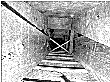
13 Existing Balcony framing conditions (existing condition)
