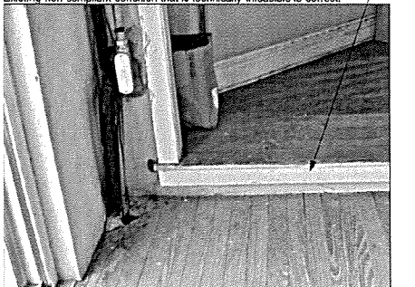
12 8" step up from Balcony to Anteroom (existing condition)
